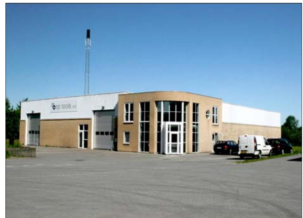
EP Tools new Facility in Denmark enables the service that our Scandinavian customers deserve and expect
